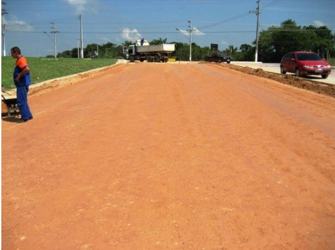
Urban pavement base in the city of Manaus, the Amazon state capital. Built with the chemical soil stabilization technology, with ECOLOPAVI -Soil Stabilizer.
